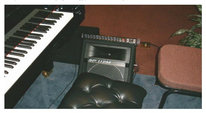
A piano floor wedge monitor is shown with a MyMix14 mounted on top of the monitor. The output jack on the rear panel feeds backstage to the piano monitor amplifier allow the pianist to listen without having to wear headphones but still able to control their monitor mix. When the musician is through playing pushing the mute switch mutes that monitor feed to the amplifier eliminating the audio in the now unneeded piano wedge monitor.
